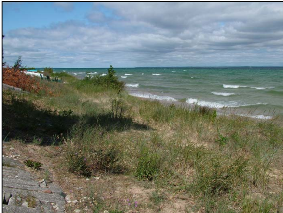
Top Photo: Slope to beach stabilized with cement blocks
